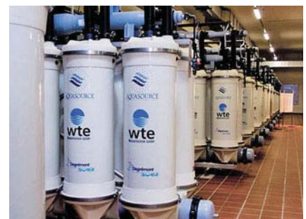
Yugo-Zapadnaya drinking water plant's purification membranes (Aquasource)
